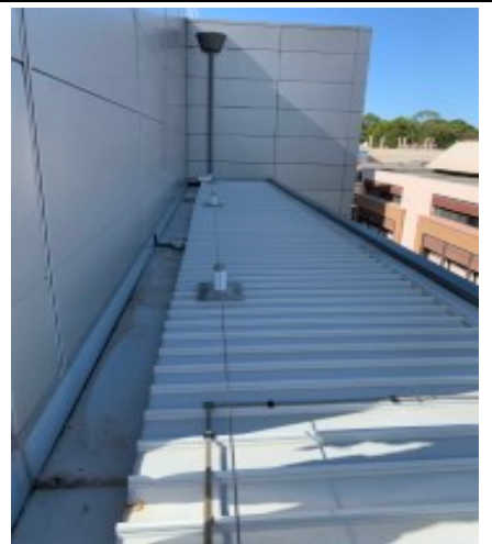
Main Roof area with lifeline (Certification by Riverlands Roofing Status Current)
