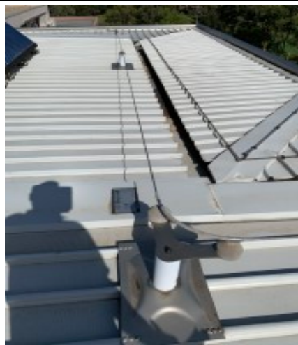
Main Roof area with lifeline (Certification by Riverlands Roofing Status Current)
