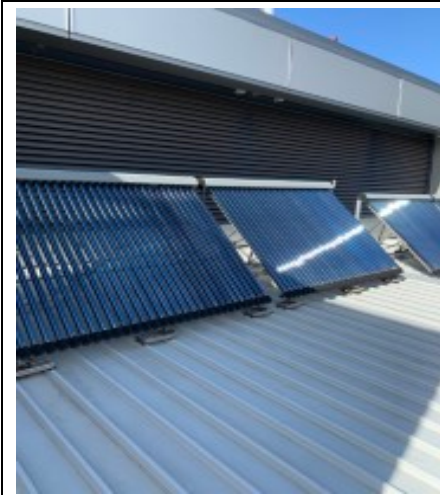
Main Roof area with solar hot water system
