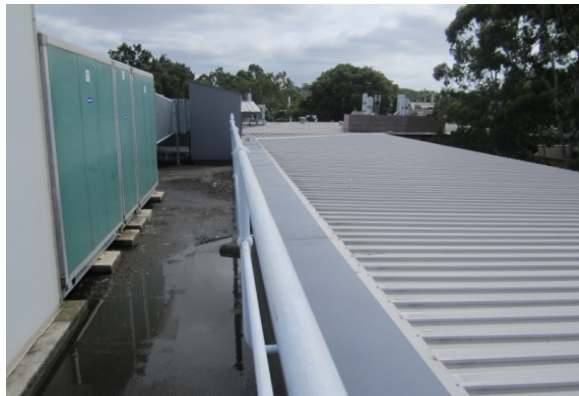
Library - Eastern balcony looking north
