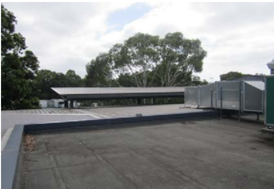
Looking North onto balcony on northern side of building
