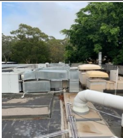
Building 2 roof area with ducts and exposed pipework
