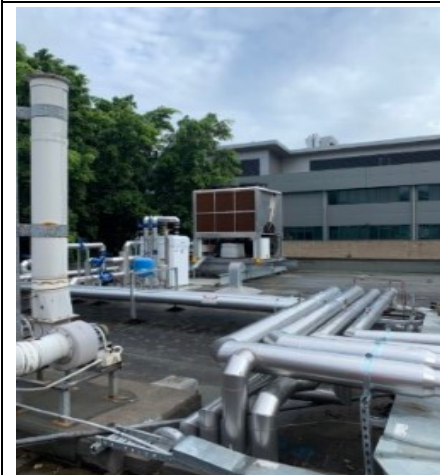
Building 2 roof area with exposed pipework & services
